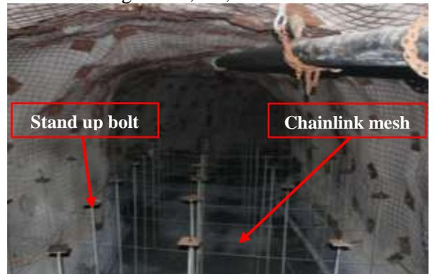
Figure 5.7. Pastefill reinforcement with the installation of chainlink mesh and stand up bolts before recharging.
