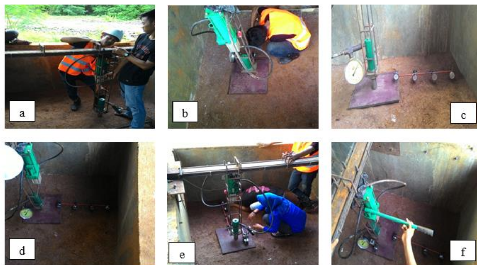
Figure 2. Model testing procedure; a) installation of test apparatus, b) dial gauge installation, c and d) hydraulic setting, e) dial reading, and f) loading test
